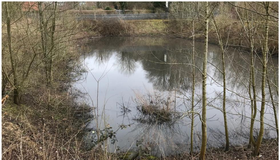
Here the proposals show modifications to the balancing pond to create a hierarchy of treatment seeking to maximise pollution removal before discharge to the publically accessible Wild Park treatment and infiltration basins. The concept plan shows the following features:
