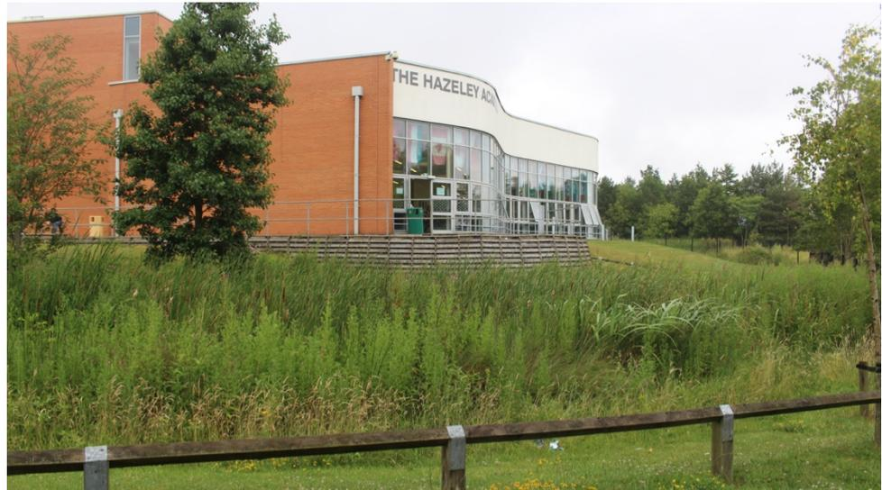
For peace of mind, an outlet from the final basin could be connected to the existing soakaways. Although these offer far less infiltration potential compared to the basins, if the modified flow route is connected back to this existing destination, it would avoid the possibility of being accused of making the drainage situation worse.
